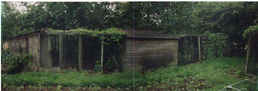
Pictures taken in the mid 1990s when the original Shelter was derelict. Above shows the scale and layout of the Main Shelter with communal run and several shed inside the communal run. Below shows the separate block of 3 kitten pens. Everything was very "make do and mend".
